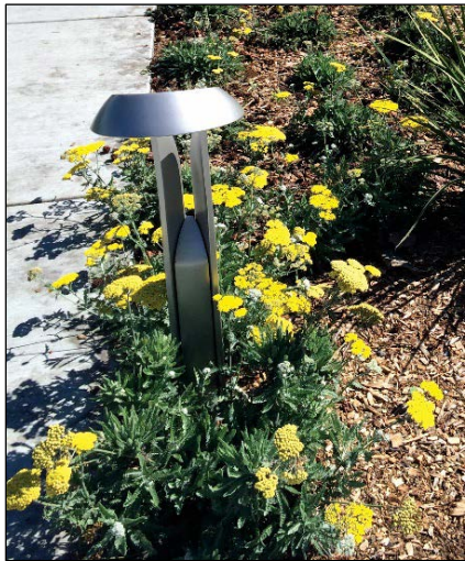
Photo 30. Bird-Safe Light Fixture that Points Light Downwards
