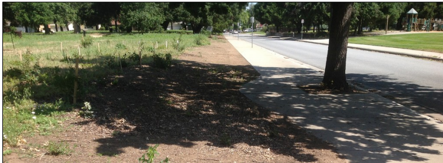
Photo 10. Sidewalk along Thousand Oaks Drive beneath a Valley Oak (This Sidewalk could be Pulled Back from the Tree into the Adjacent Meadow to Protect Tree)
